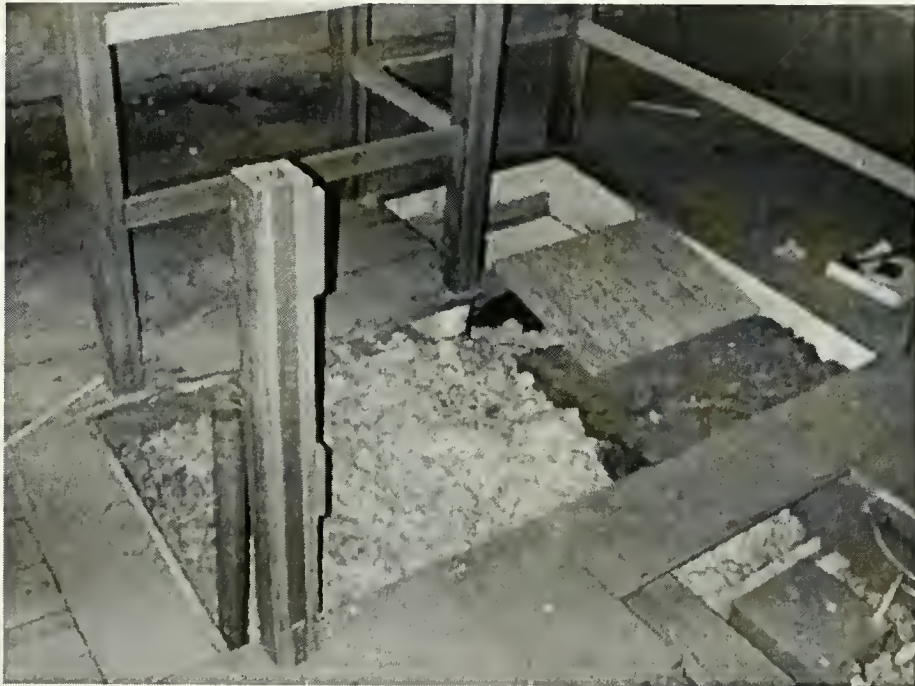
Figure 39 Third generation Stair Opening in Attic of Center Section of the Main House, 2002
